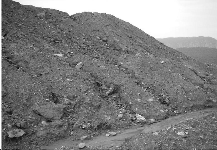
Figure No 10. The view of the slope at the waste dump (water seepage related sliding observed at few locations)
