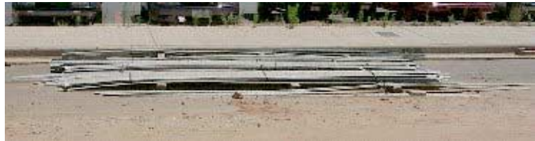
Figure 15, Reinforcement Storage
