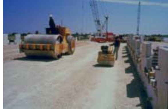
Figure 21, Compaction Equipment
