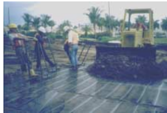
Figure 38, Tensioning Polymer Reinforcement
