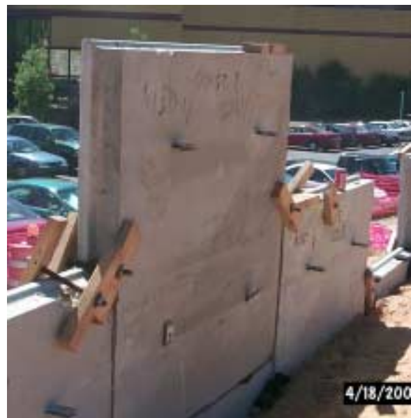
Figure 11, Damaged Tabs
