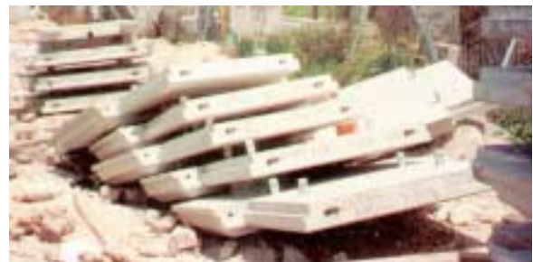
Figure 10, Improper Panel Storage
