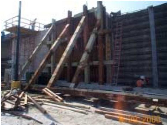
Figure 30, Temporary and Permanent Wall Facings
