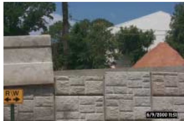
Figure 16, Leveling Course for Coping/Barrier
