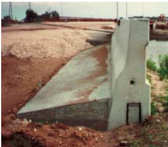
Figure 17, Barrier with Slab
