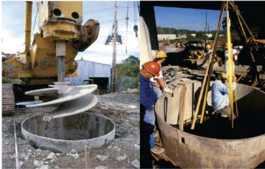
Figure 4-6 Drilling into Rock through a Cased Hole
