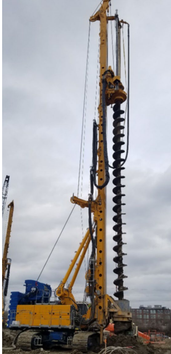
Figure 7-1 CFA Piling Rig (photo by authors)
