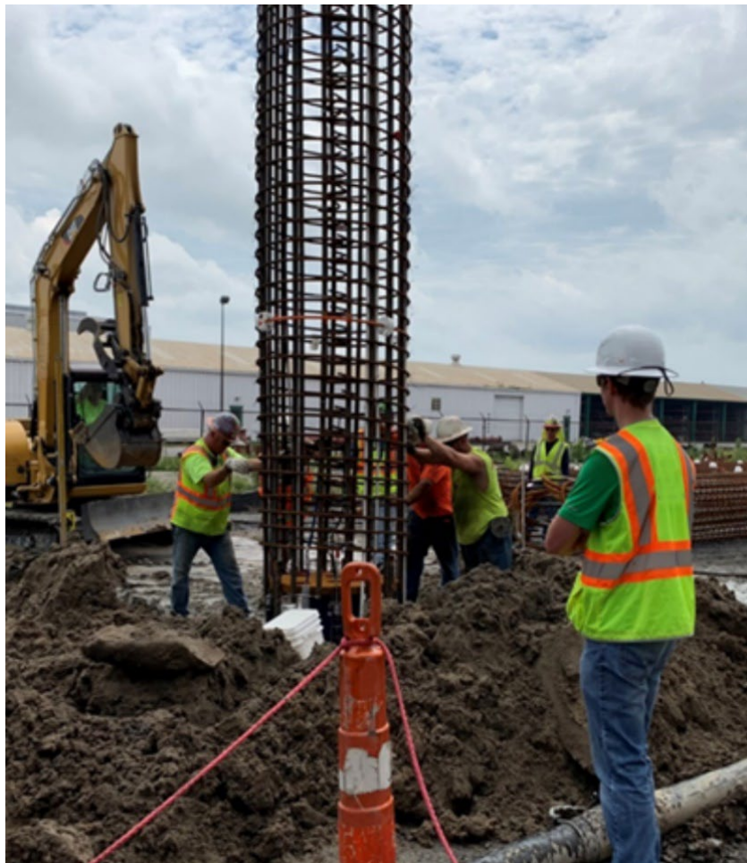
Figure 7-2 Placing Reinforcement in a 48-inch diameter CFA Pile (photo by authors)
