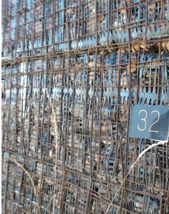
Figure 20: Flexible facing with a wrapped geogrid connection
