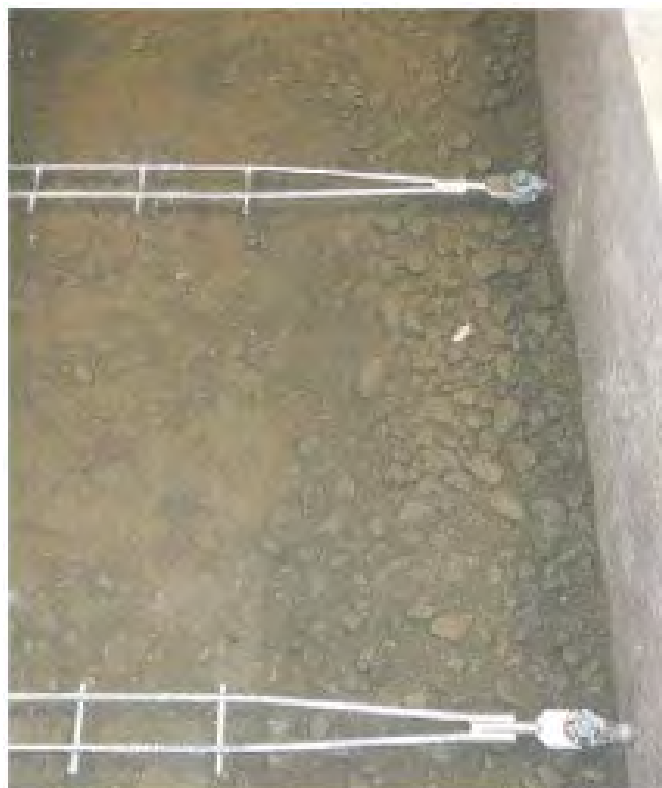
Figure 12: SCP and two-wire steel strip reinforcement connection
