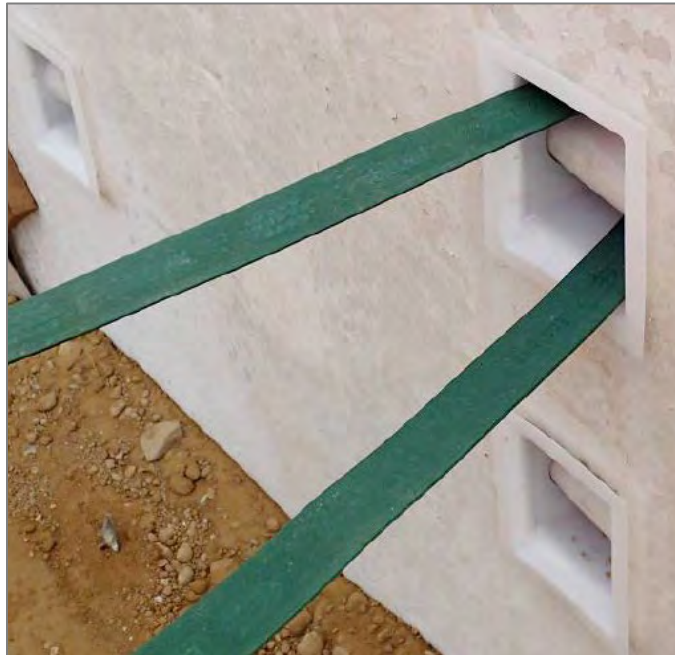
Figure 15: SCP and geosynthetic strip connection
