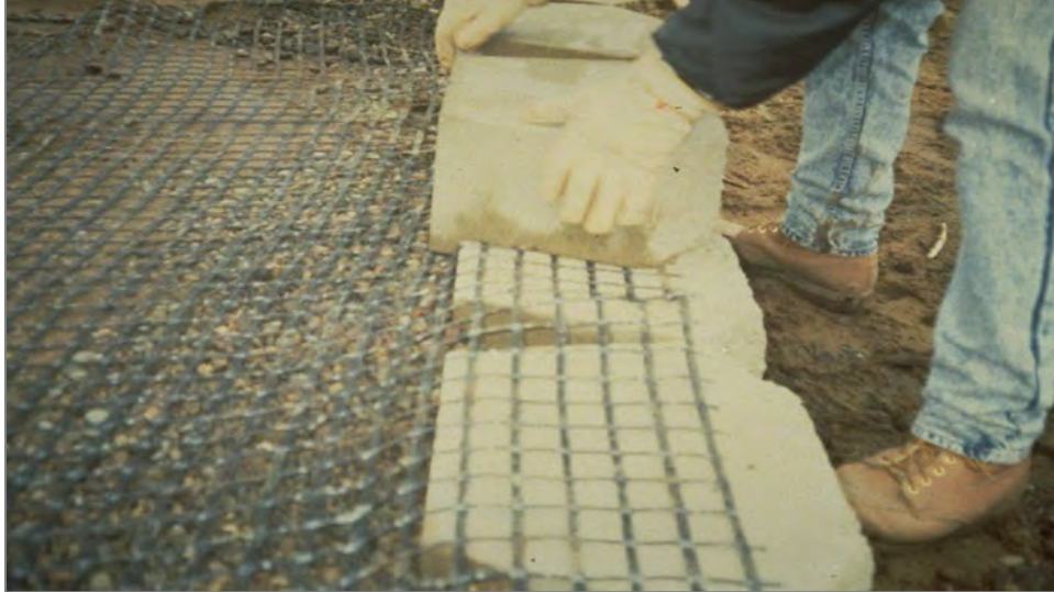
Figure 16: MBW unit and geogrid frictional connection
