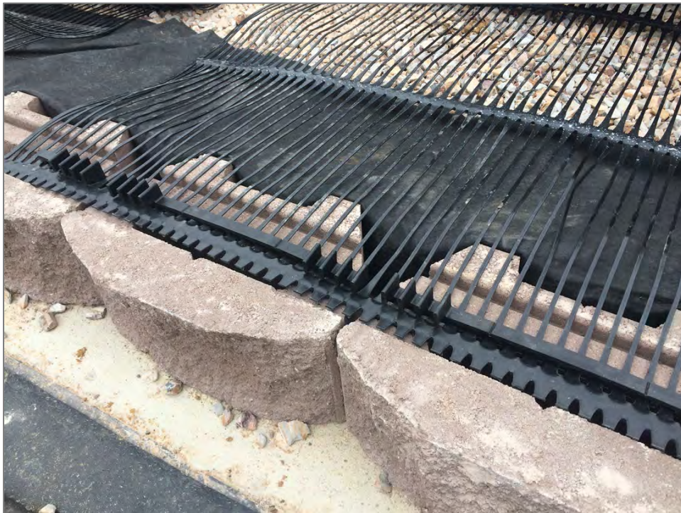
Figure 17: MBW unit and geogrid mechanical connection
