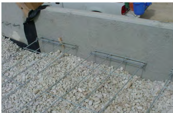
Figure 13: SCP and steel wire grid reinforcement connection
