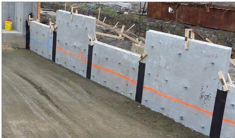
Figure 22: Geotextile filter on SCP
