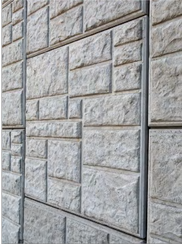
Figure 7: SCP facing (Courtesy RECo)
